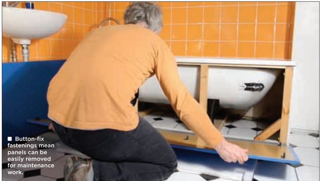
■ Button-fix fastenings mean panels can be easily removed for maintenance work.
